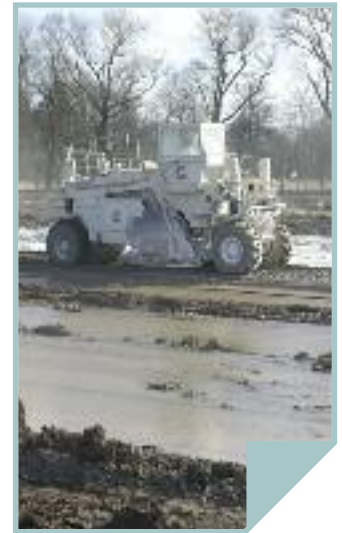
Conditions were far from ideal when stabilisation was started.
