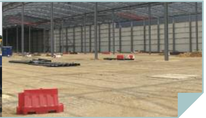
Below: After flooding, Firmaroc still provides a strong, safe platform for cladding erection. After steel/cladding Firmaroc still remains intact and free from rutting.
