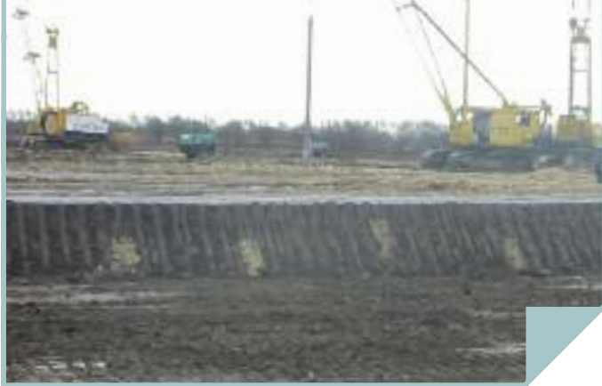
Above: Vibro piling rigs using Firmafil as piling platform.
