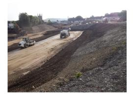
This was a subcontract for Thomas Armstrong Construction to undertake ground improvement works to a maximum 9m depth below a housing development. The site was a former gas works on significant slope and involved the excavation and deposition with *Firmafil* treatment of 9,000m3 of on site material and the same treatment to 8,000m3 of imported materials. The site also had significant areas of localized pits which were also successfully treated
