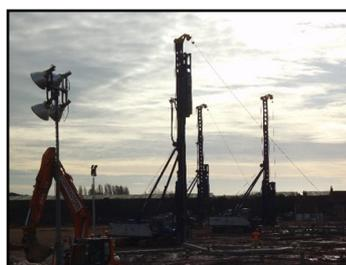
Upon completion of the Firmafil works to formation level the top 300mm layer was Firmabase stabilised to 30% CBR and topped off with 75mm stone. This acted as the piling mat for up to four piling rigs.
